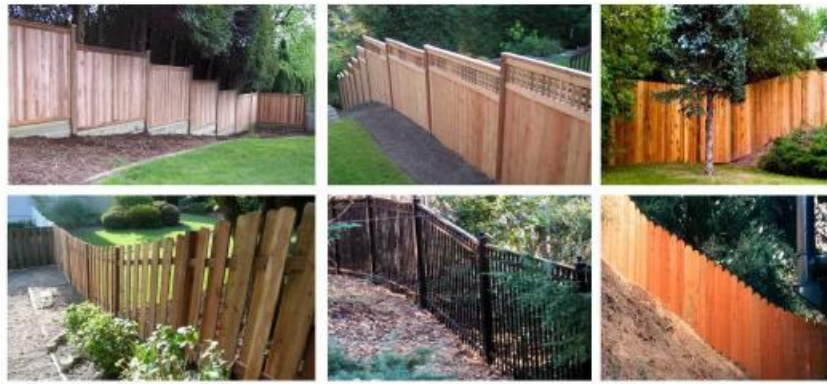
Figure 11: Fences on slopes.
