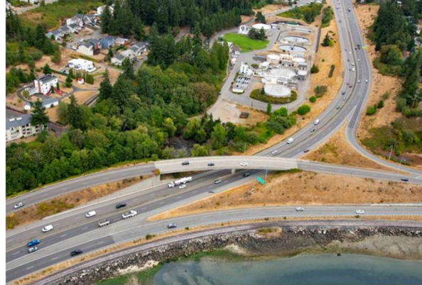
Charleston Boulevard overpass at SR 3.
