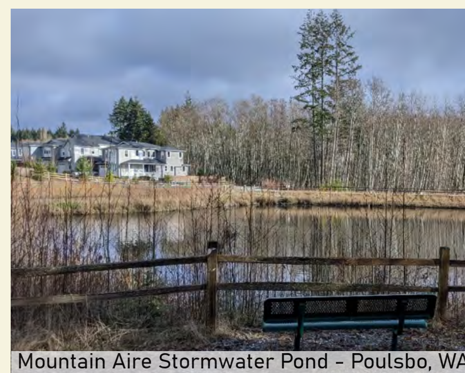
Mountain Aire Stormwater Pond - Poulsbo, WA
